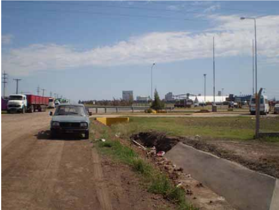
Ingreso Area Industrial
